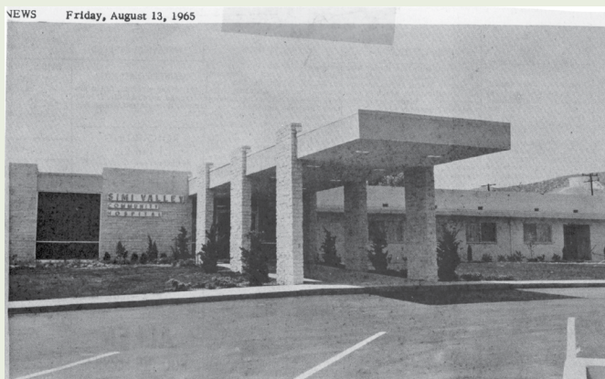
THE 50-BED Simi Valley Community Hospital which will hold its open house, dedication and formal opening on Sunday, August 15, at 2 p.m. Located at 2975 North Sycamore Drive, Simi, the hospital is the first to be built in the Simi Valley.
