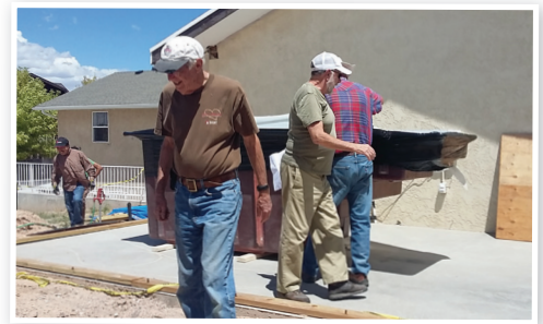
Cedar City church members work on a new baptistery.
