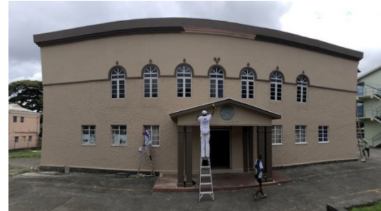
After: building is completed with a fresh coat of paint.
