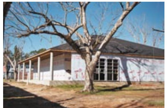
Practice rooms in the music building have become recognizable as drywall is hung.
