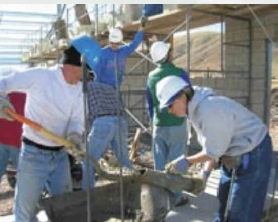
Florida Hospital DeLand team members building a new elementary school.
