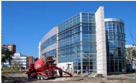
New sidewalks are poured next to the campus center.
