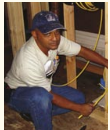
Aaron Wildman, a licensed electrician, runs wires for an electrical outlet.
