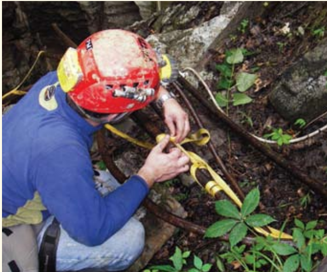
After removing the pipes from the cave entrance, Southern graduate assistants untied the webbing used to pull them up so they could be hauled away.
