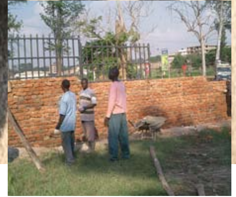
UNIFAT's partially completed fence
