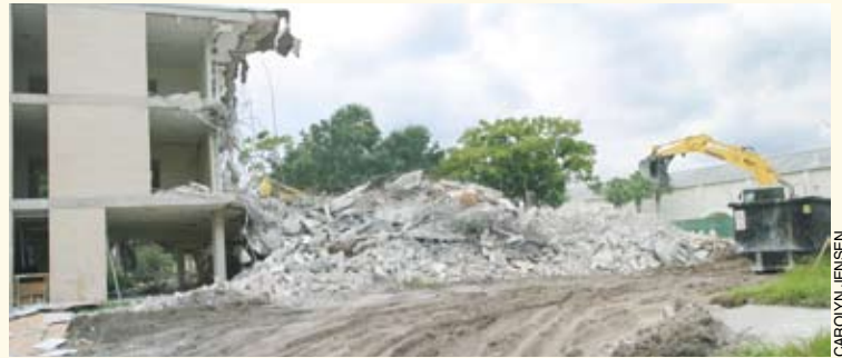
Demolition workers clear away 44-year-old McClure Hall.
