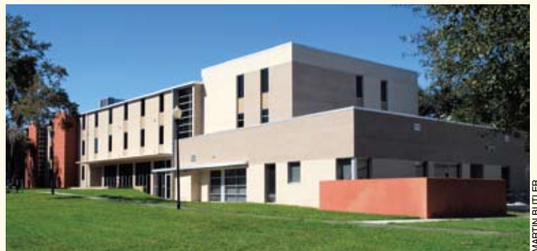
The old girls' dormitory east/west wing was converted into McClure Hall (pictured with expansion) for male residents. The renovated north/south wing still serves as Memorial Hall for female residents.
