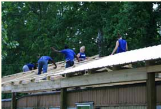
Members of the team put the roof on a pole barn to cover a member's trailer home in Monticello, Ky.
