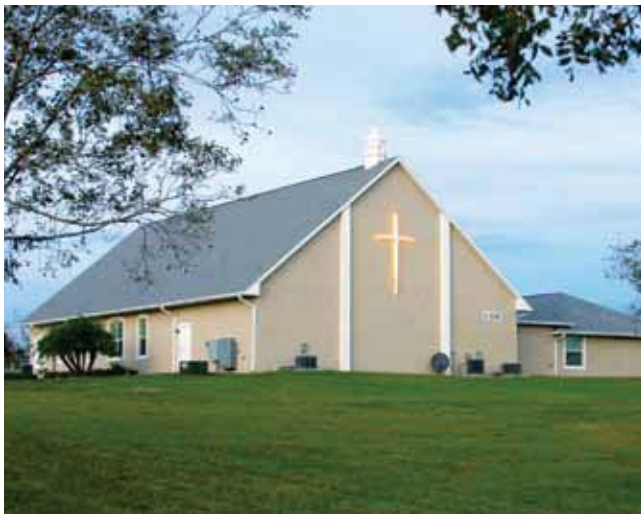
The North Lake congregation built its new church facility on five acres of land near Umatilla, Fla.
