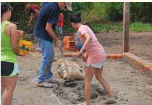
David Denton and Coleen Moralde mix the cement by hand.
