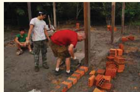
Andrew Jamieson (center) and crew build the church.
