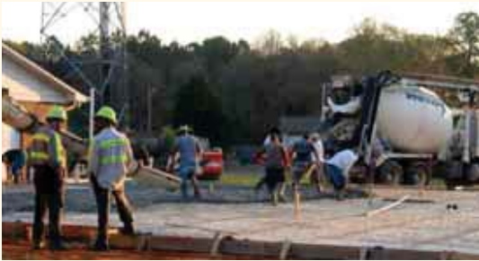
Loganville Church sanctuary foundation being poured. The church celebrated the opening of this new sanctuary on August 20, 2011.
