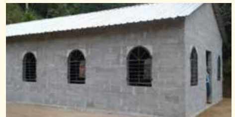
Less than two weeks after groundbreaking, the new Cerro Campana, Panama, Church is ready for occupancy.
