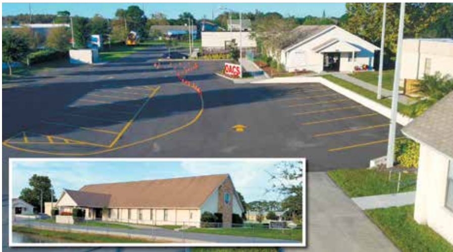
Members and guests gathered on the Kissimmee Church and Osceola Adventist Christian School campus to celebrate the completion of structural improvements, and express gratitude to individuals who gave their professional skills, financial support, and encouragement.
