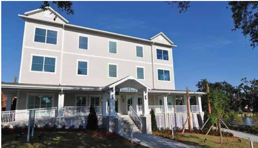
The Bartch Transplant House features 24 private rooms, a kitchen, laundry facility, and common spaces for families of transplant patients.
