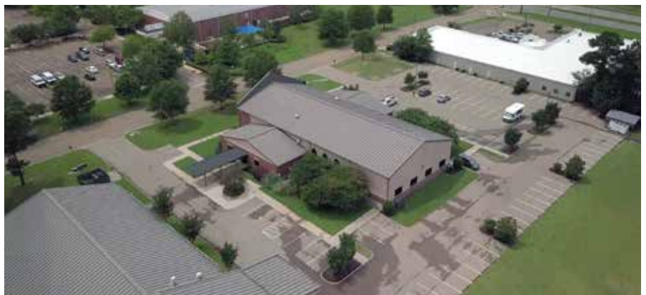
The church will expand its main building to the east in order to accommodate the growing ministries.
