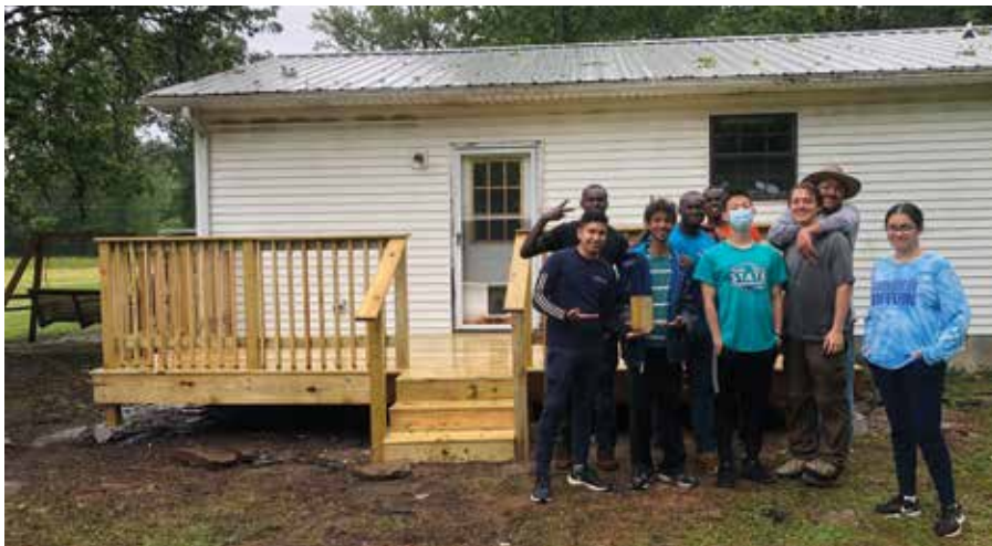
A group of students restored a deck.
