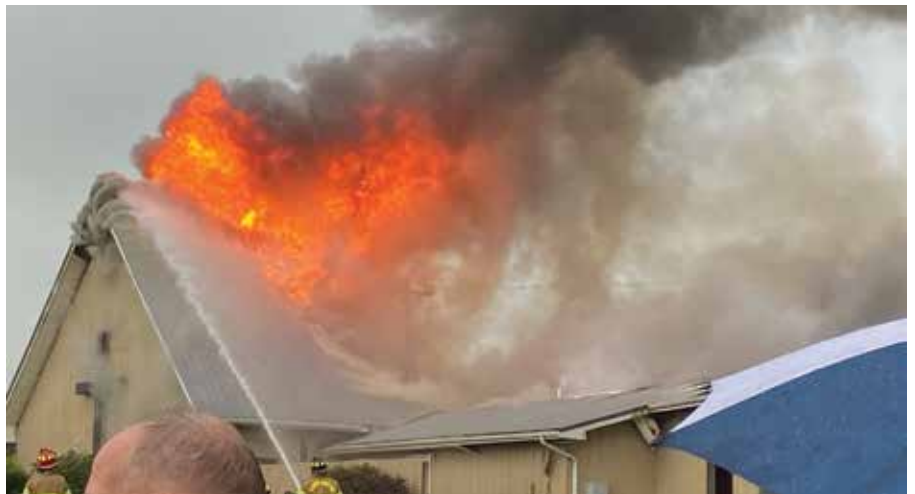
The Riverview Community Church in Greeneville, Tennessee, was hit by lightning and burned to the ground on August 17, 2021. Members are meeting at a nearby church they had rented from Riverview nearly 30 years ago when they were needing a place to worship.
