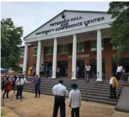
Peterson Hall and University Conference Center is a $7 million renovation.
