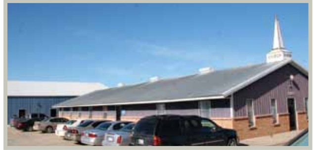
The new addition to the Woodward church, which was recently dedicated.
