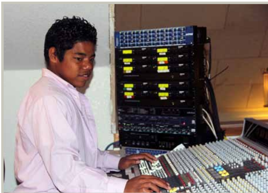
Danny Heim operates the Springdale church sound system.
