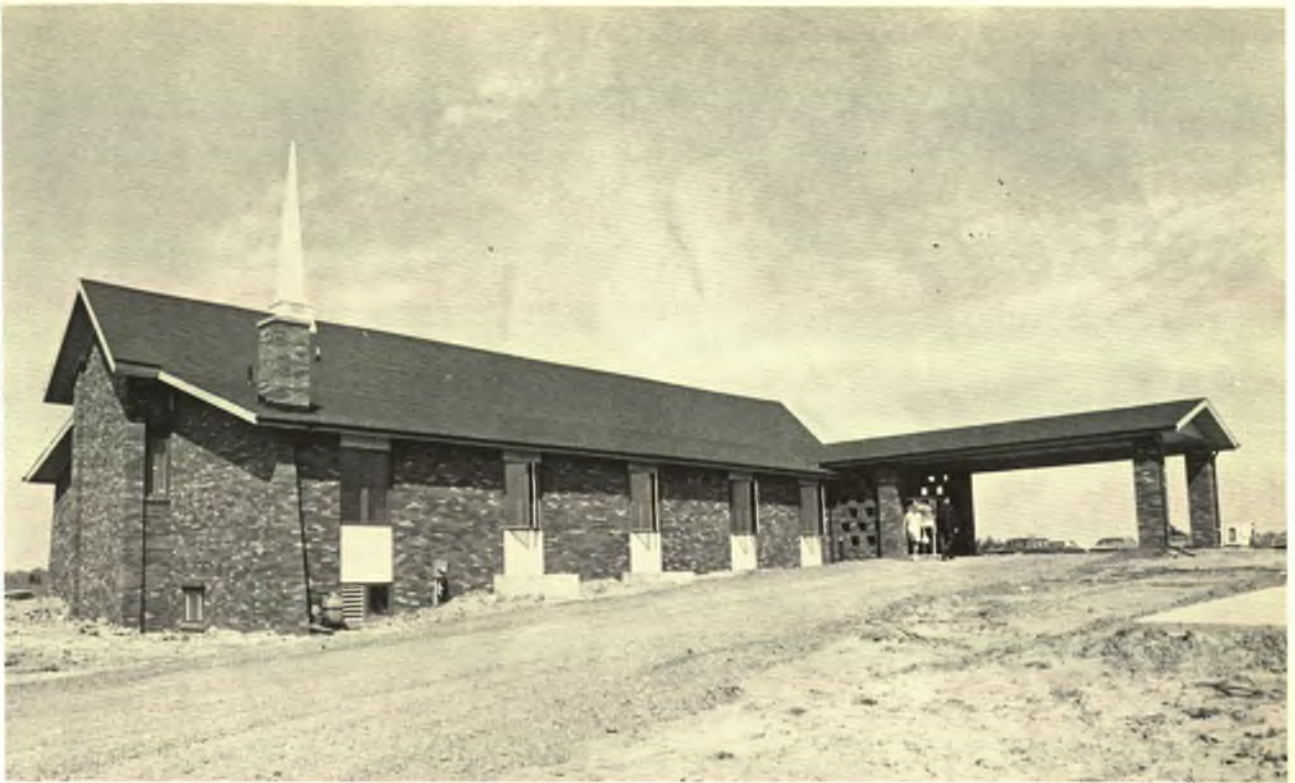
Exterior of the Adrian Church on opening day.
