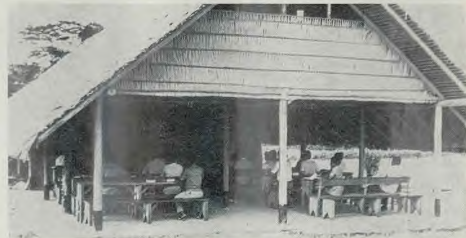
One of the first classrooms built on the school site and which has served many purposes. Timber and thatch from the school property have been used since the beginning of the school to economize in the building programme.
