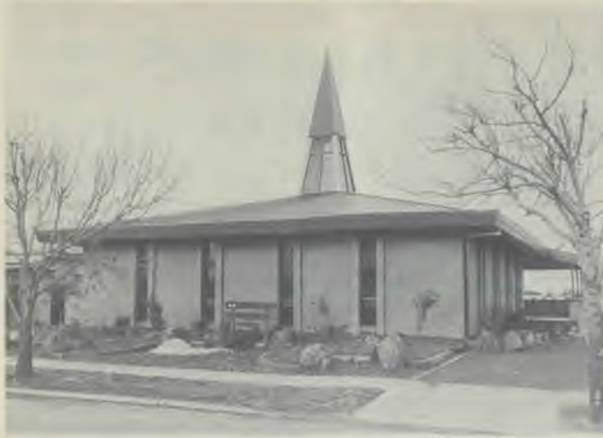
A new sanctuary. Solid and appealing, this structure is a testimony to the practical efforts of its members.
